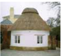
New Forest creamery. Before and after reconstruction, using cob blocks made from the collapsed material.
