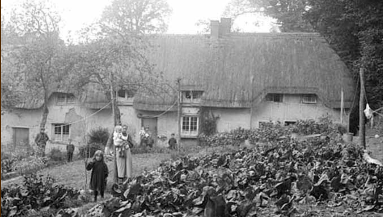
Right: Cob cottage, Outwick, near Fordingbridge. Some render is failing on front of cottage.
