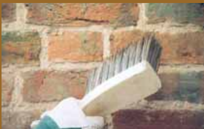
The surface of the mortar can either be profiled to match an existing style, such as double struck, or "jointed" with a jointing tool, or it can be given a "weathered" finish by washing with mist fine spray or by tamping with the bristle ends of a churn brush, further compacting the joint. Brushing should never be applied across the mortar as this leaves unsightly drag marks. Wet sponging should never be used as this leaves lime deposits on the bricks and stones which become obvious as the work dries out.
