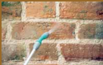
The surface of the mortar can either be profiled to match an existing style, such as double struck, or "jointed" with a jointing tool, or it can be given a "weathered" finish by washing with mist fine spray or by tamping with the bristle ends of a churn brush, further compacting the joint. Brushing should never be applied across the mortar as this leaves unsightly drag marks. Wet sponging should never be used as this leaves lime deposits on the bricks and stones which become obvious as the work dries out.
