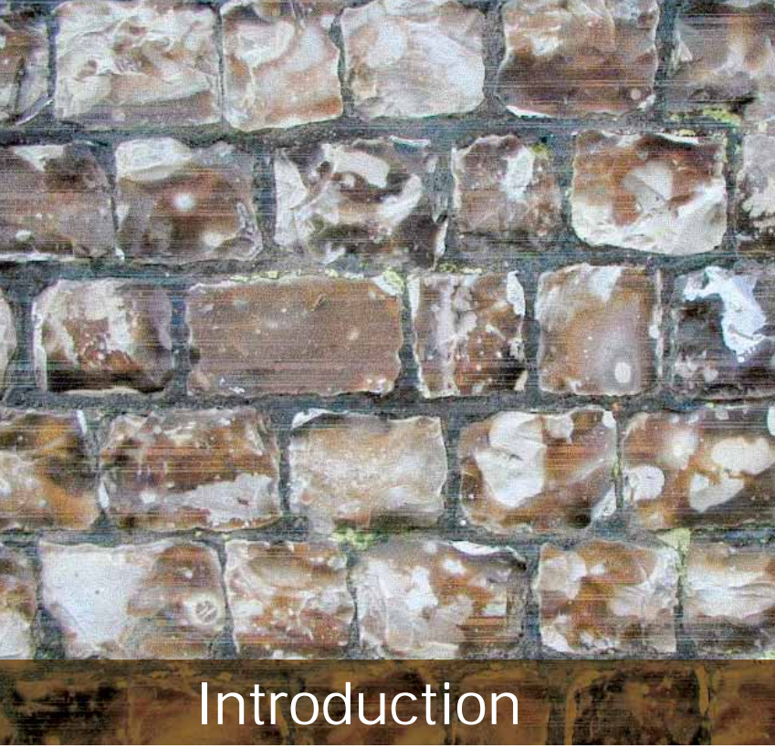
ABOVE: Shows tabular flint in a black ash mortar gauged with oil.
