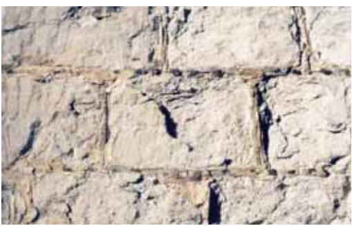
Shows the soft grey malmstone from the north-east of the county with sandy, yellow lime joints and dark garstone “nails”, often referred to as galletting.
