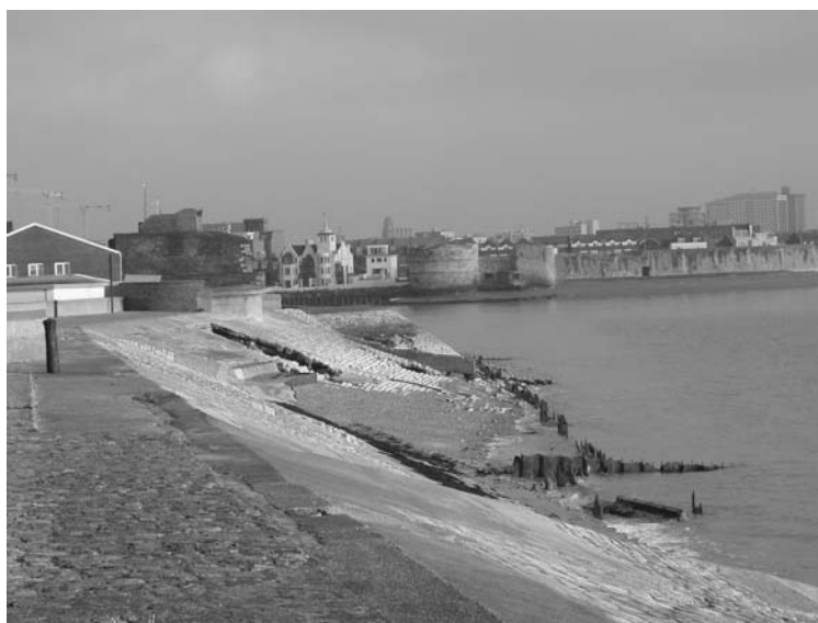
Fort Blockhouse, Gosport looking towards Old Portsmouth defences. Future sea level rises and storm surges will increase coastal flooding and place many structures at risk if predictions are accurate. (Archaeology SE-UCL)
