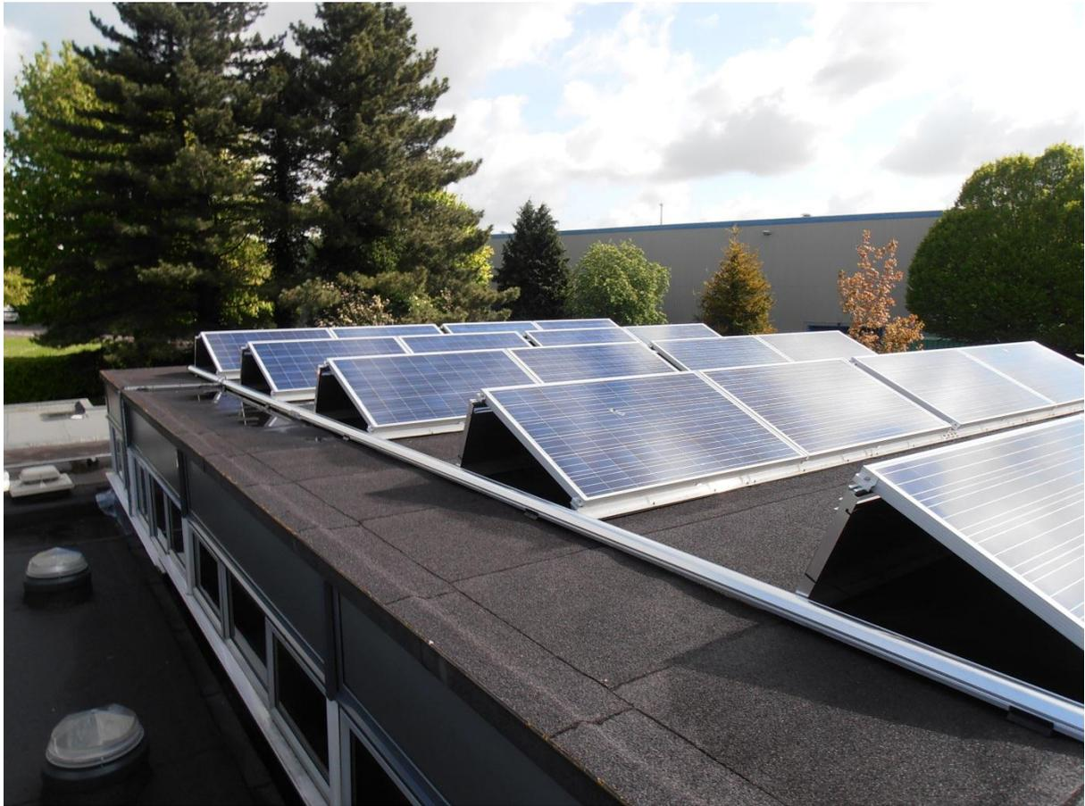
**Image 3: Finished installation on the roof of Icknield School.**
