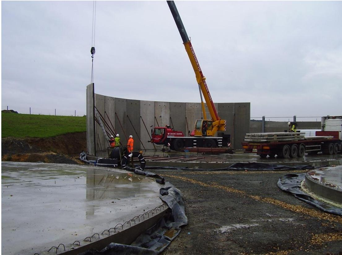
Fig 2.0 Segmental concrete tank construction showing leakage membrane.
