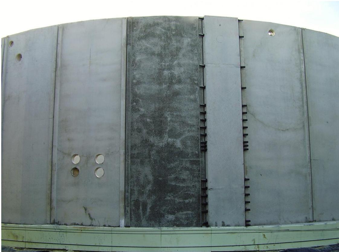
Fig 1.0 Buttress Panel showing cable ends on segmental constructed tank.
